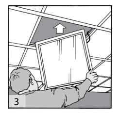
The light panel is being lifted through the hole in the ceiling system.
